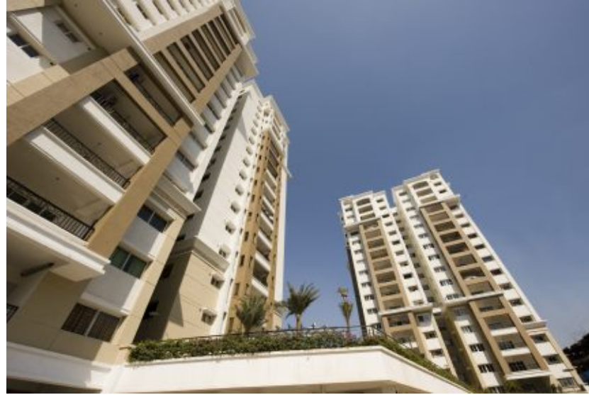
FORTUNE TOWERS, Madhapur
